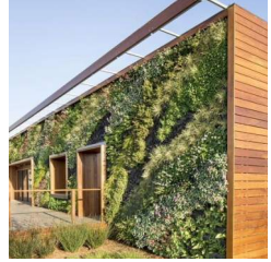
VEGETATION WALL LOCATION: PATIO
